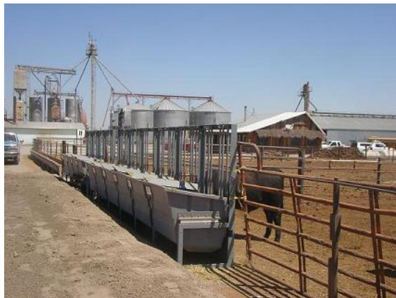
FIGURE 1. Snyder Livestock Sire Testing Facility, Yerington, Nevada
